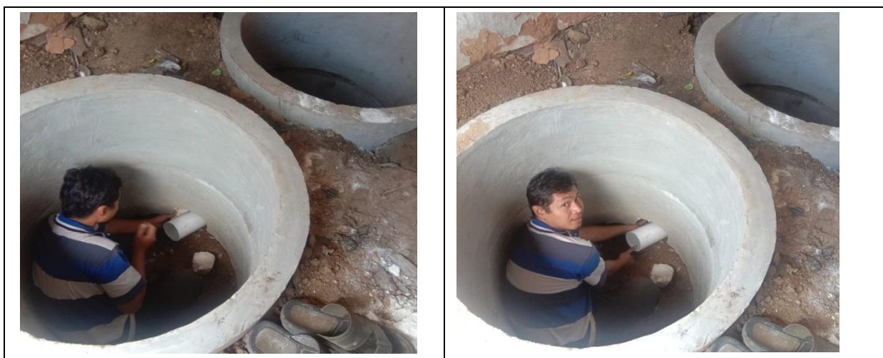
Figure 12. Installation of biogas pipes
