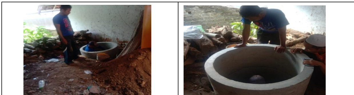
Figure 11. the process of excavating the soil and laying Tampolong
